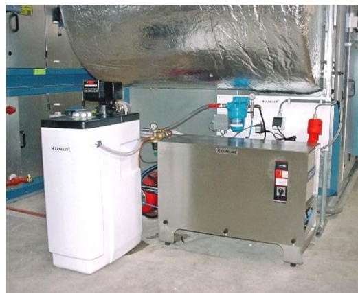
Ontharder 12, filter en Combi-Compact®
